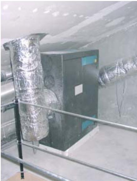
Ventilation unit with heat exchanger in the building services floor of a Hannover-Kronsberg Passive House. In the background is the fresh air duct with defrost heater and in the foreground is the exhaust air pipe (both insulated with mineral wool, aluminum laminated)
